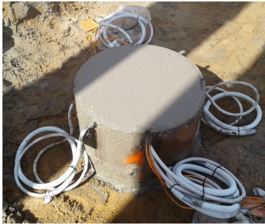
Figure 6 A pile head and the sleeved FO cables at the exit points
